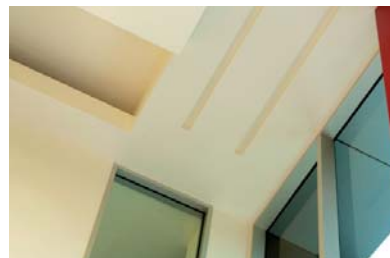
Studco Fastcap used to create a feature rebate in a ceiling.
